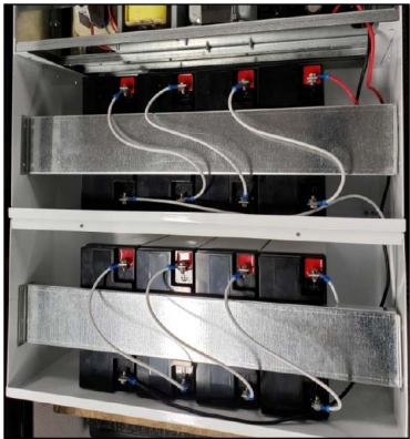
Battery brackets installed on the front
